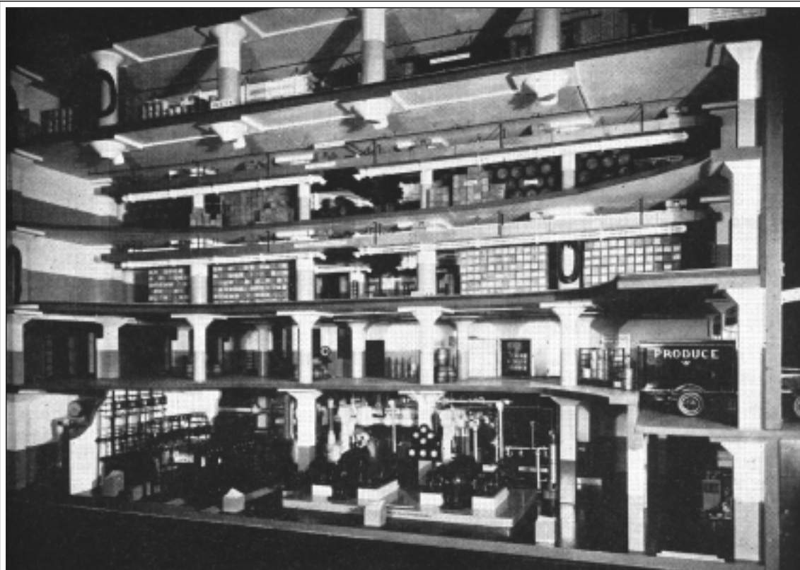
A true to scale model of a cold storage plant with more than 2,000 individual castings was conceived by an ASRE committee and built by Berthold Audsley in 1931. The model showed the insulation, refrigerating system, elevators, and power plant equipment. The model was loaned to the Chicago Museum of Science and Industry.
